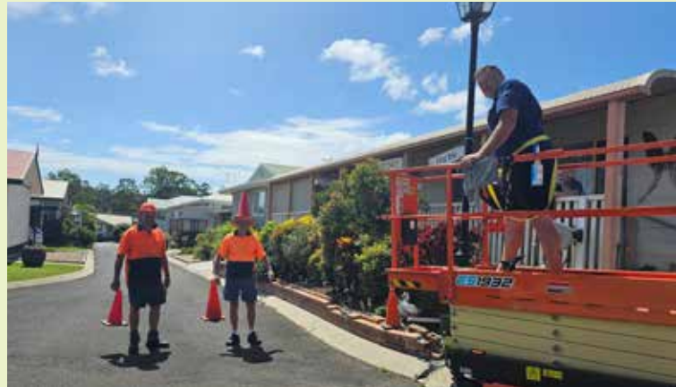
Pictured above: We snapped Caretaker Wayne fixing the lighting around the resort, with the help of David, our Groundsman, and Stuart (Home 168). The trio were rewarded with coffee, cold drinks and ice creams!
